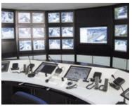
was designed and installed by the Company's local Approved Partner Cyberguard Systems for the Municipal Council of Penang Island. The system consists of 31 PTZ dome cameras connected via a wireless IP network monitoring the whole of the Georgetown area. The cameras are focussed on crime and traffic hot spots such as tourist areas, banks, petrol stations, traffic intersections and commercial centres. www.indigovision.com
