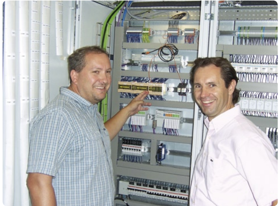
Rolf Gasser (40) and Markus Schönbächler (47) in front of the control cabinet of the FS 680 filling machine. The only 22.5mm wide safety module Vital (right) allows to connect different safety devices.
