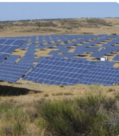
◀ Abertura Photovoltaic Solar Plant spans a surface of over 200 hectares. More than 132,000 solar panels on 2,112 solar trackers with a total installed power of 23.1 Mega Watt peak.
