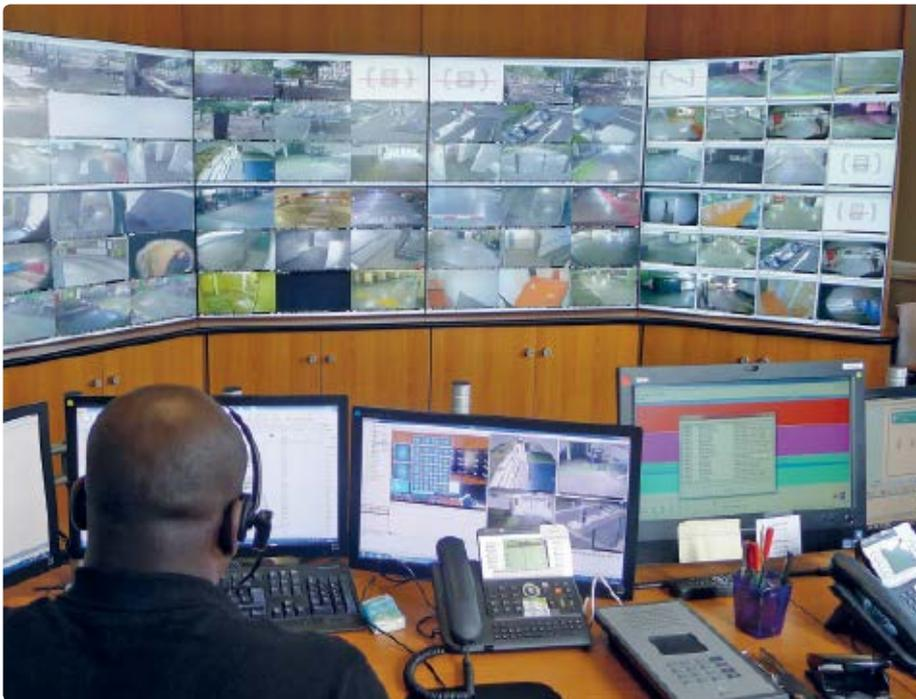
From this central location, the control room staff respond to all service requests and emergency calls from the clients in the car parks, so no human presence in the car parks is actually necessary. To visualize the CCTV camera signals, Eyevis has installed a 7m<sup>2</sup> video wall, consisting of twelve 46" type EYE-LCD-4600-M-USN-LD displays. The incoming signals are controlled by a Netpix 4800 graphics controller and the Eyecon wall management software.
