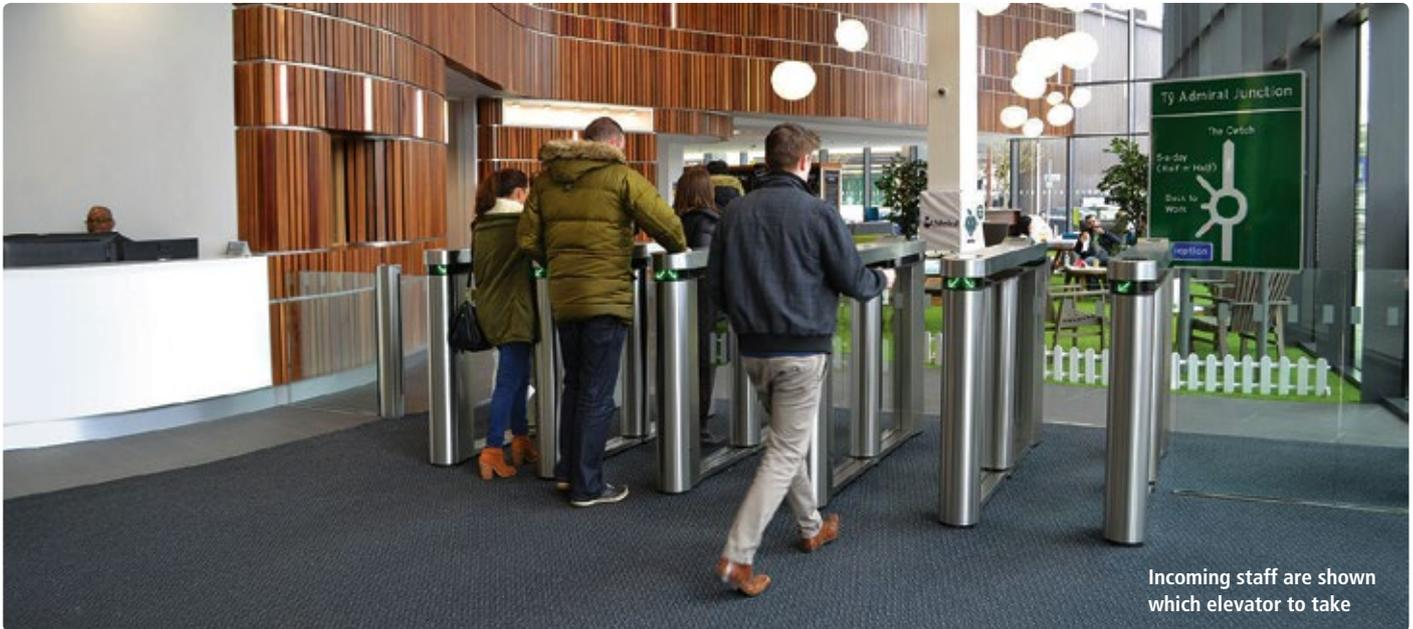
Sovereign Fire and Security has recently completed a building management system at Ty Admiral in Cardiff. The new access control and elevator destination system reduces time spent by staff queuing and improves the efficiency of people getting to their work floor. The system, which has been developed together with TDSi and the elevator manufacturer Otis, is the first one of its kind in the UK.
