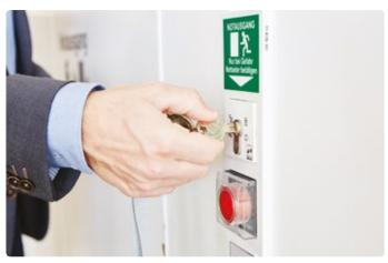
The key switches integrated in the emergency exit control terminal permit switching the door to permanently open state
