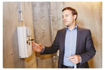
The key safes, among other locations also installed in the lift lobbies (here in a surface-mounted version), allow an electronically secured removal of the key and provide a reliable fall-back
