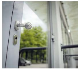
The flush form of the door cylinder prevents damage
